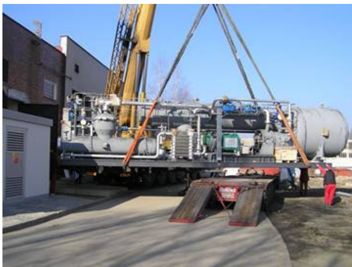
Obr.5 - Instalace modulu ORC
